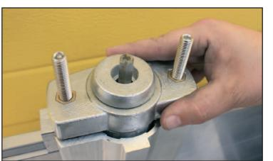
1 When using the demountable post, secure each post by using the 10mm socket and torque wrench provided, by turning the top central hexagon, clockwise, until the post is firmly secured to the ground.
