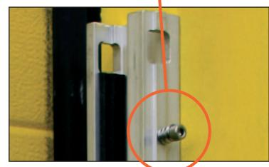
5 Twist demountable post, clockwise, 90-degrees into position to accept the flood board, with the cap head screws facing outwards, the same face as the vertical side channels. Note – there is no need to tighten the posts in place at this stage.
