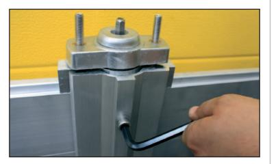
**7** On the front face of the vertical side channels, by hand, start turning the horizontal 10mm grub screws, clockwise, until they are finger tight.
